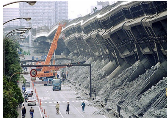
Fig.1 Higashi-Nada Viaduct collapse in 1995 due to Kobe earthquake [3]
